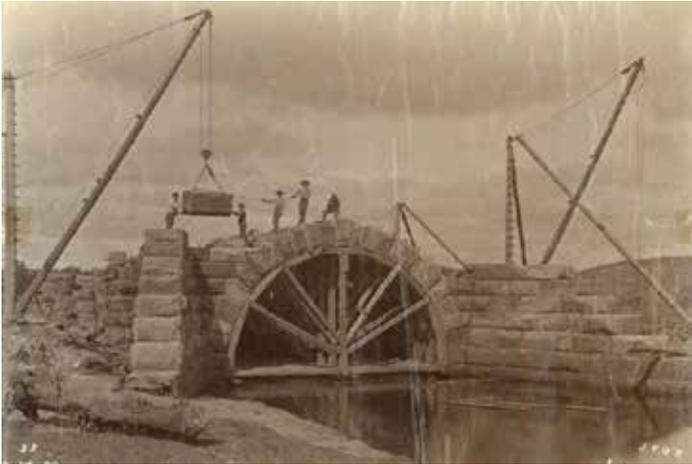
Engineers directing the building of a stone culvert. Dave Rathfon, *The Story and History of the 1864 Stone Arch Culvert Railroad Bridge*, [www.backtobradford.com](http://www.backtobradford.com).
